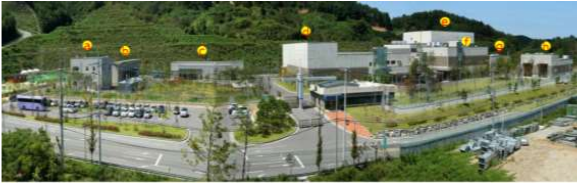
Fig. 2. Layout of the surface facilities; a) Waste Water Treatment Building, b)Garage, c)Equipment Maintenance Shop & Warehouse, d)Radioactive Waste Receipt & Storage Building, e)Radioactive Waste Treatment Building, f)Service Building I, g)Service Building II, h)Power Supply Building
