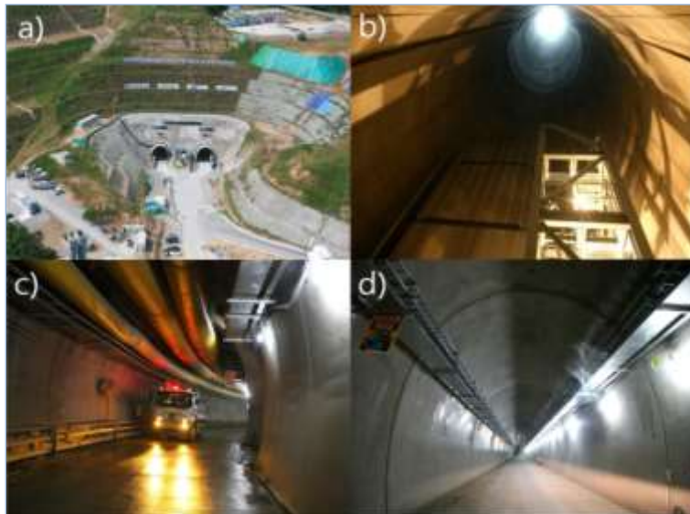
Fig. 6. The view of Construction ; a)Portal, b)Shaft entrance, c)Operation tunnel, d)Construction tunnel
