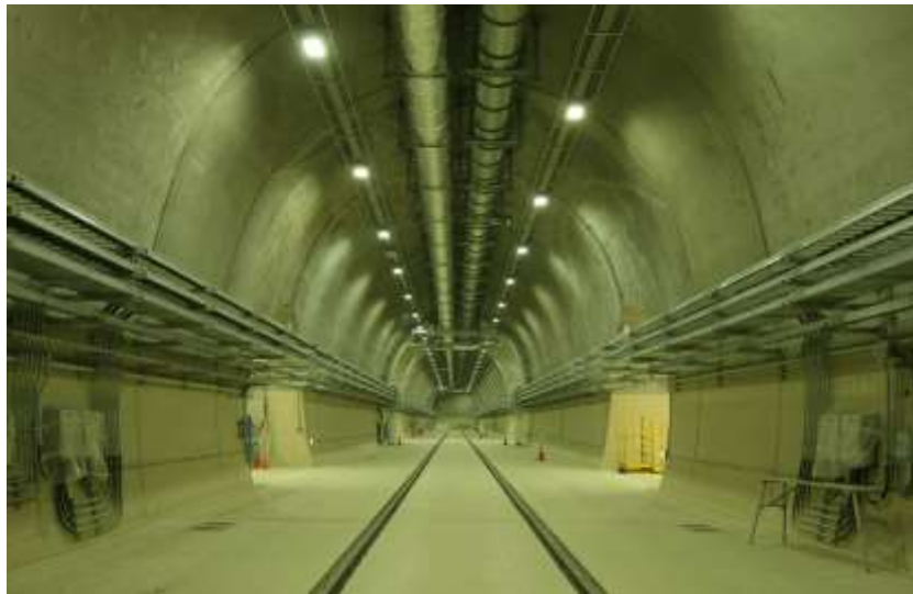
Fig. 9. The view of unloading tunnel
